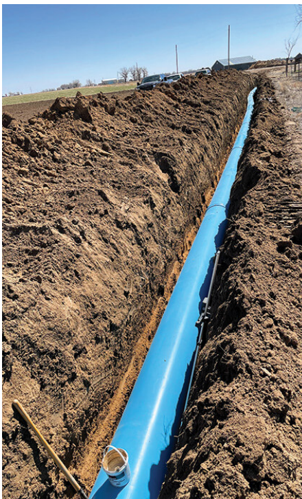
Installation of the center pivot system at MB3 Farms. Photo credit Irrigation Today.
